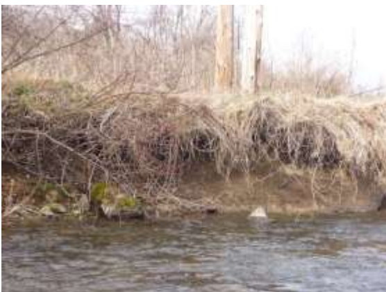
Upper Milesburg Erosion
