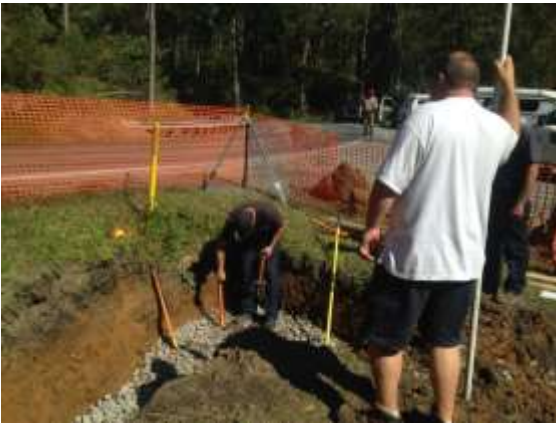
Building the diverter
