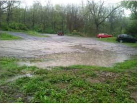
Rock Road Before Improvements
