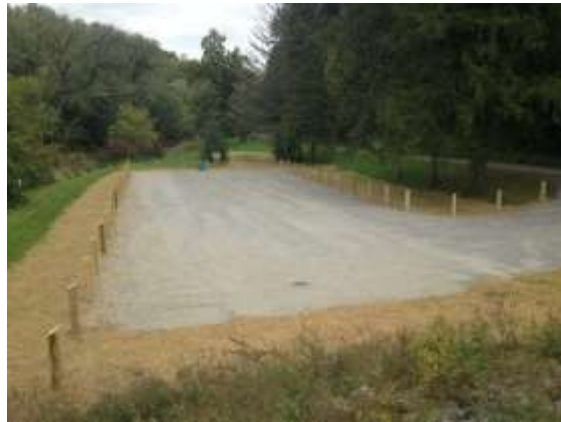
Fisherman's Paradise – Lower parking lot. Stormwater diverted to swale on right away from creek.
