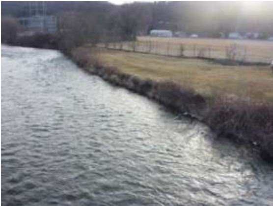
Lower Milesburg Project – 2012 Before Note –Step Bank, No Plant, mowing to edge
