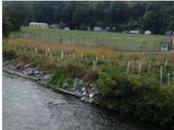
Lower Milesburg – September 2014 200” Mudsill protecting bank, native trees and shrubs, wildflowers and interpretive sign.
