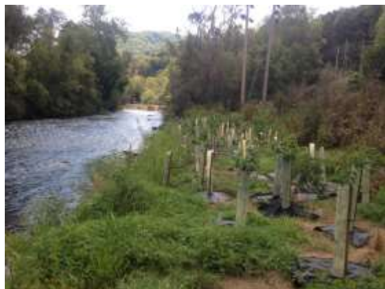
Upper Milesburg – After 4 multi-vane log deflectors, coir log, and riparian planting.
